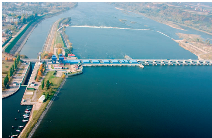
Fig. 1. Włocławek barrage – view from the upstream side
